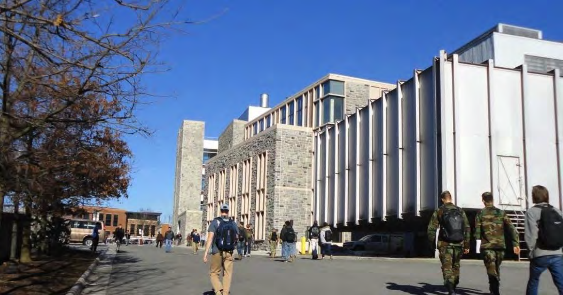
Service corridor behind Durham Hall
