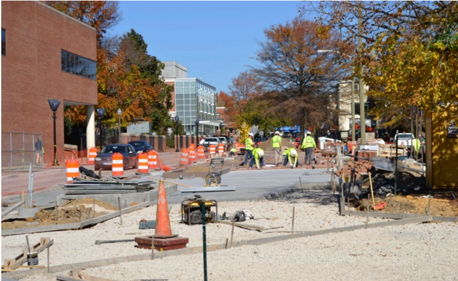
College Ave. Promenade Substantial Completion: July 2013
