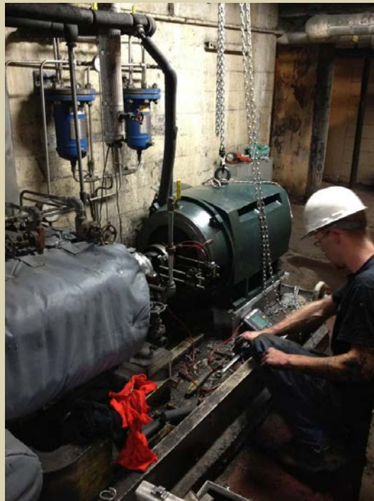
Powerhouse Insulation Blankets
