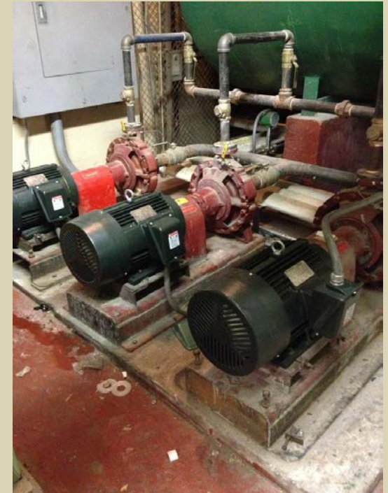
Powerhouse Inverter-Duty Motors (for future Variable Frequency Drives)
