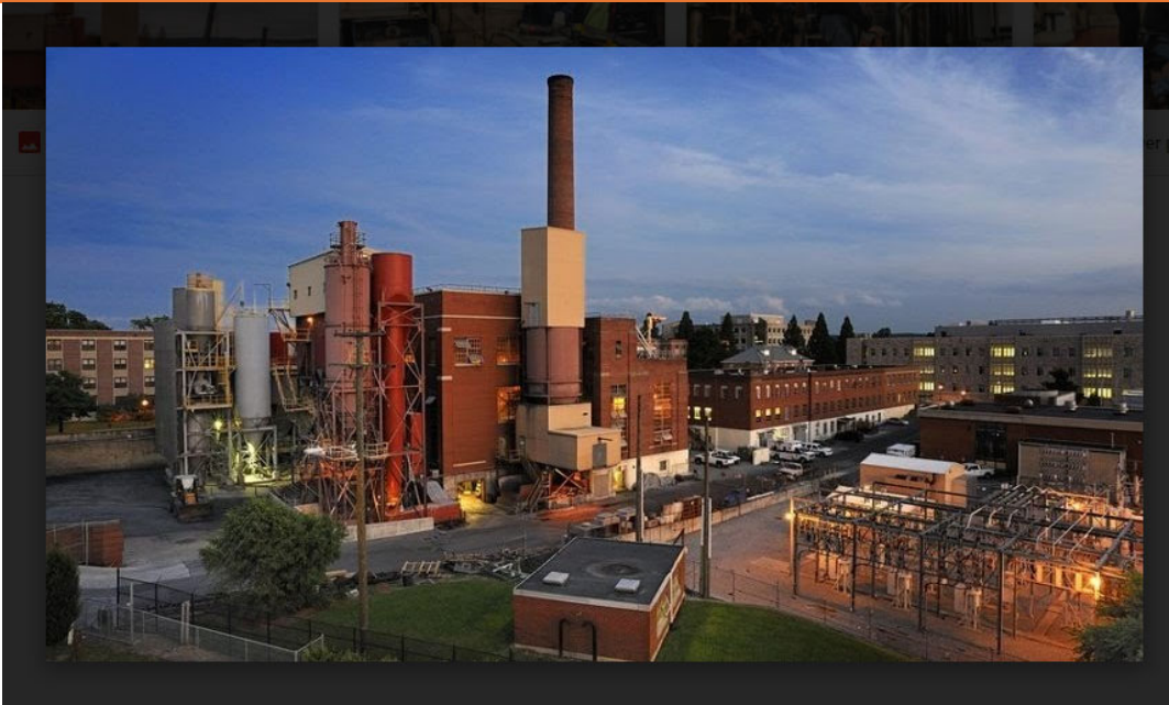
Virginia Tech Central Steam Plant, Virginia Tech Electric Service Blacksburg Substation (foreground) and the North Chiller Plant (behind substation)
